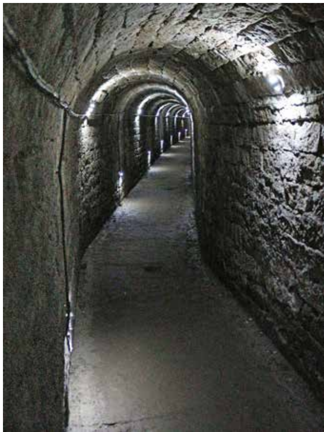
Chatsworth coal tunnel
